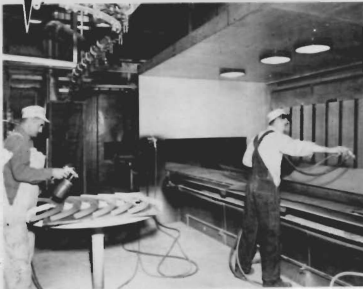
PAINTING SECTION —Complete conveyerized paint facilities for spray and dip painting.
