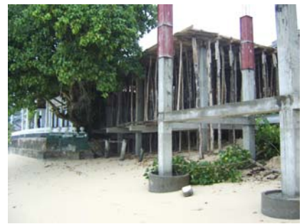
Under construction, January, 2006
