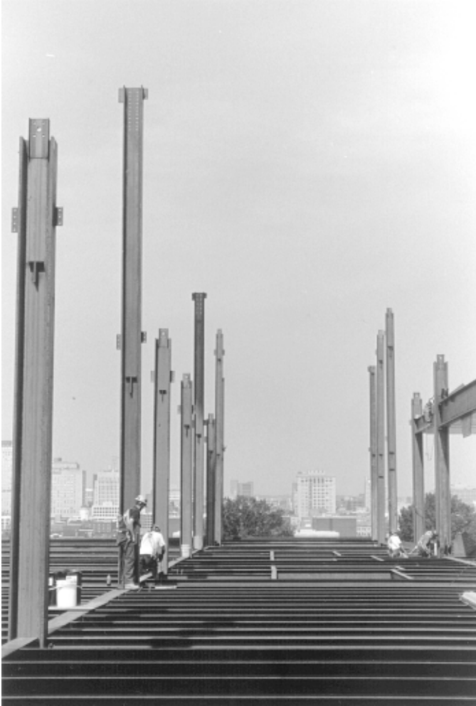
Ironworkers connect sections of structural steel.
