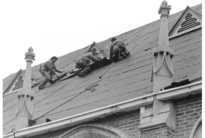
Roofing work is strenuous, involving heavy lifting, climbing, bending, and kneeling.
