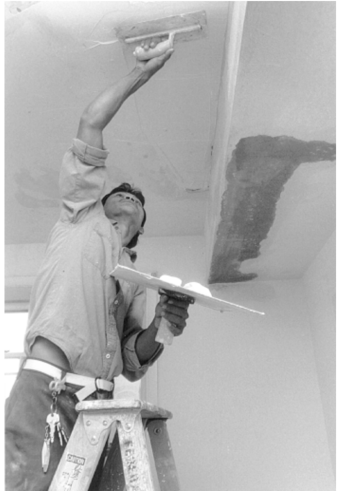
Plasterers repair old plaster and install plaster in new construction.
