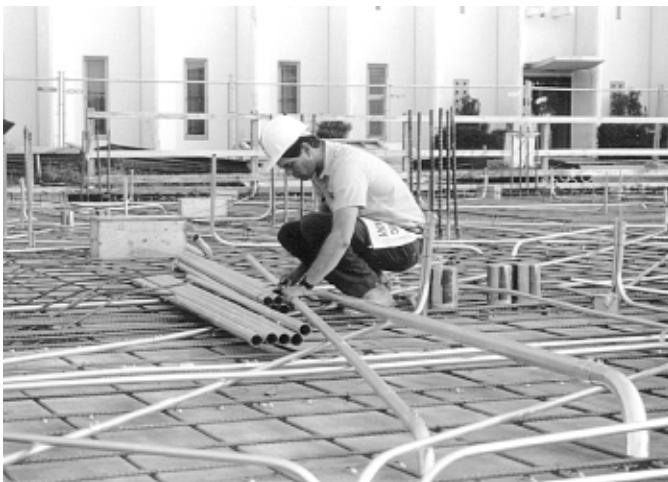
Electricians lay out conduit for electric wires.
