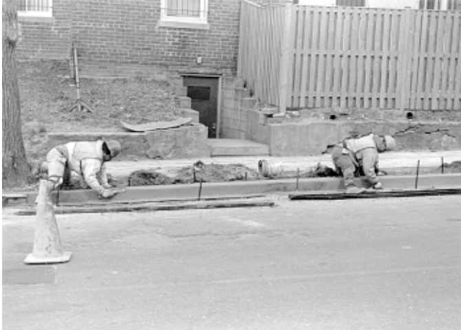
Concrete finishers use hand trowels to smooth the surface.
