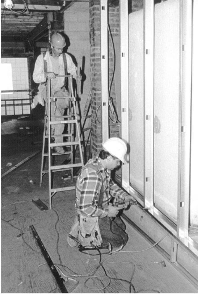
Some carpenters specialize in framing walls and partitions.
