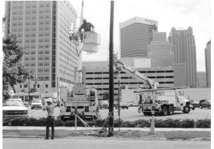
Line installers use truck-mounted buckets to reach the tops of telephone poles.
