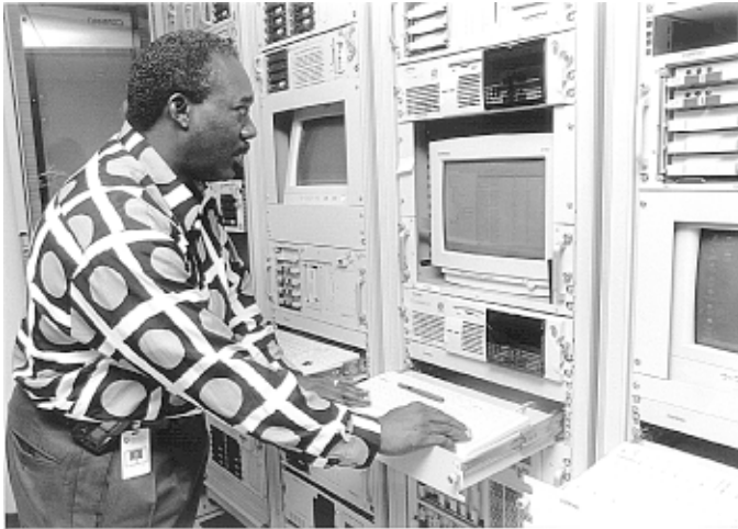
Computer hardware engineers work with circuit boards, computer chips, keyboards, modems, and scanners.
