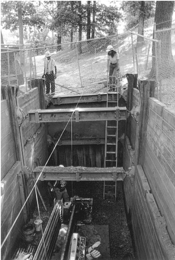
Civil engineers check on construction sites and monitor progress.
