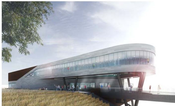
Artist's rendition of the Wellness Center under construction on campus.
